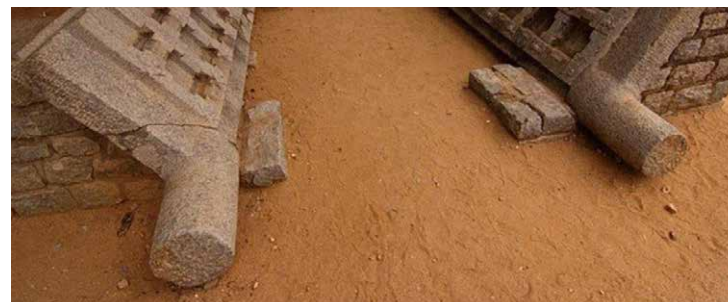
Two massive stone pivot doors in Hampi, India, where the spindles are still clearly visible. Image courtesy of Shriram Swaminathan.
